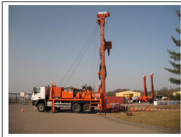
The lorry with the drill RIGG
